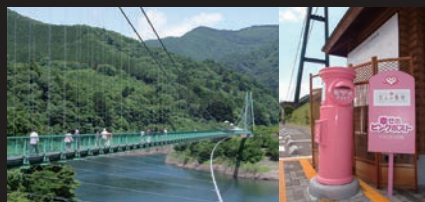
Momijidani Suspension Bridge
