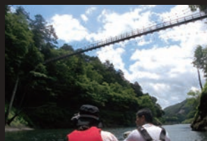
Mikaeri Suspension Bridge
